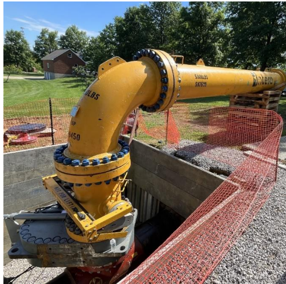
Figure 5: 24" Launcher Set-Up
